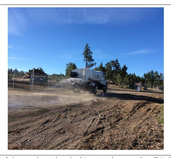
**Photo 1:** A water tender was observed applying water to the access road near Shrine Camp Staging Yard (C 440 Phase II) after the morning tailboard to minimize dust emissions during crew egress in accordance with APM AIR-02.
