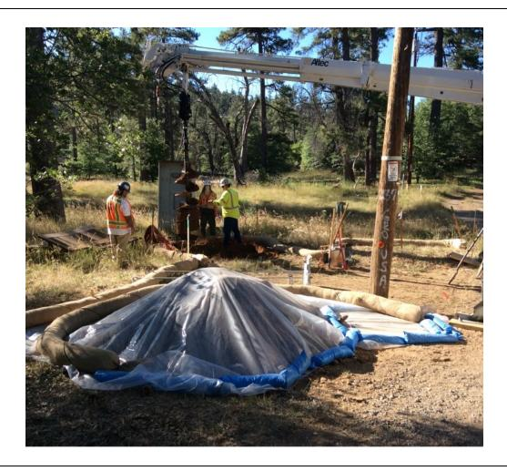
**Photo 3:** Archaeological and Cultural Monitors were observed monitoring anchor excavation and inspecting spoils for sensitive resources along C 440 Phase II in accordance with the HPMP, APM CUL-04, and MM CUL-1. In addition, the pole hole and spoils stockpile were observed to be covered in accordance with MM BIO-23, the ECP (MM HYD-1), and the SWPPP (MM HYD-1, MM BIO-7).
