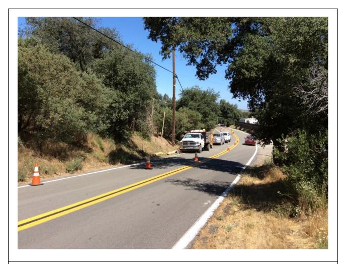
**Photo 6:** Cones, signage, and flagpersons were used to direct one-way traffic around the work area for Vault 71 and P259843 and P259844 (C 440) in accordance with the Traffic Control Plan (APM TRANS-05) and APM TRANS-02.
